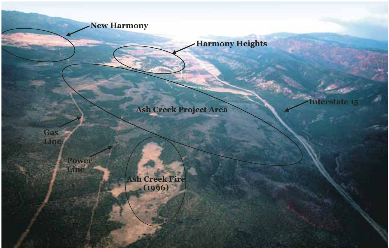
Figure 1. Aerial view of the Ash Creek project area looking northeast (posttreatment). Photo by Paul Briggs.
